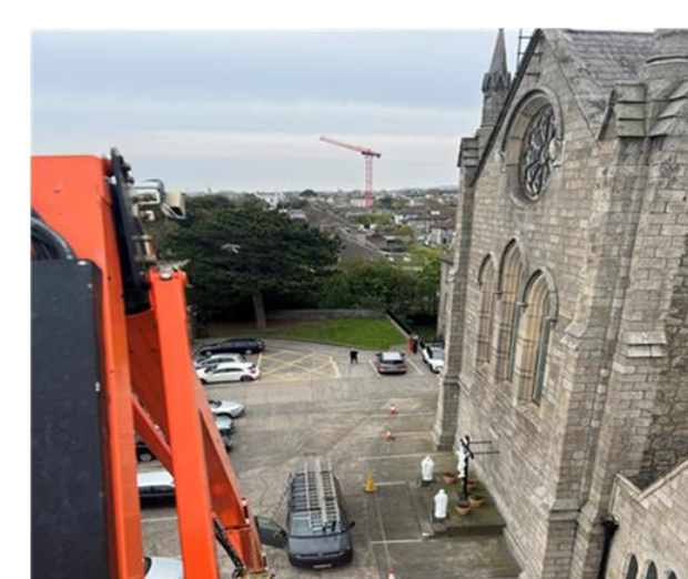
Fr. Peter inspecting the work on the cherry-picker.
